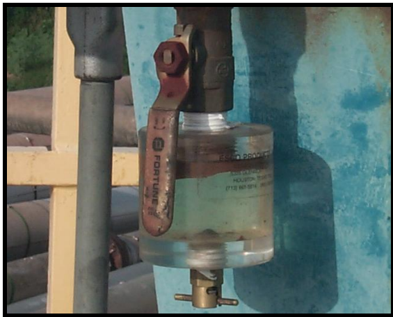
The Esco Sight Glass clearly displays water that is in the oil system.
