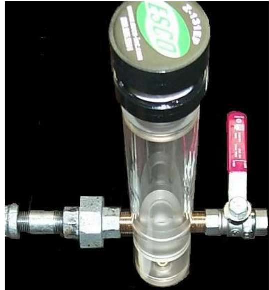
Using a Union Allows for Proper Vertical Alignment without over-tightening
